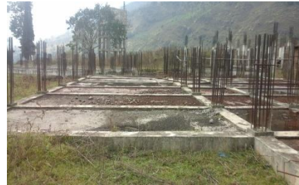
Construction up to plinth level done
