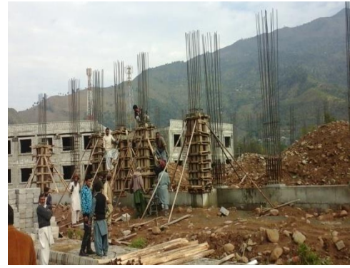
Steel fixing and concreting in progress
