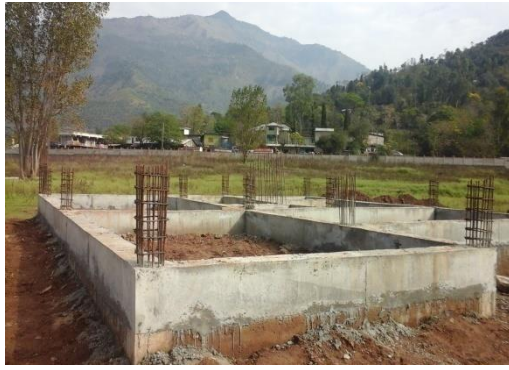
Construction work up to plinth beam done
