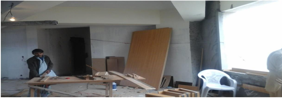
Carpenter busy in wood work for cupboard
