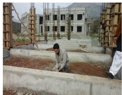
Concrete strength being checked with concrete testing hammer
