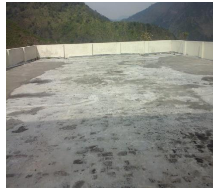
Roof treatment not done yet
