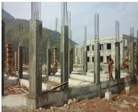
Watering/curing being done
