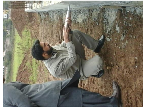
Concrete strength being checked with concrete testing hammer
